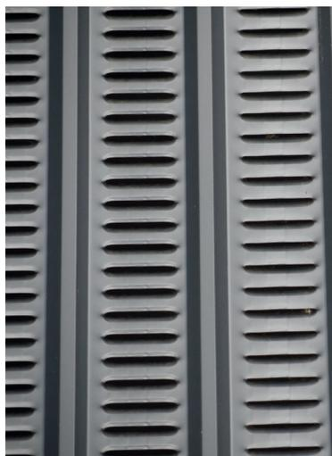
**Figure 7: Louvered cladding (18% void area)**
