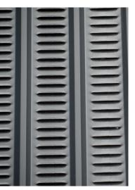
*Figure 7: Louvered cladding (18% void area)*
