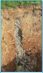
Permeable backfill in trench over drain
