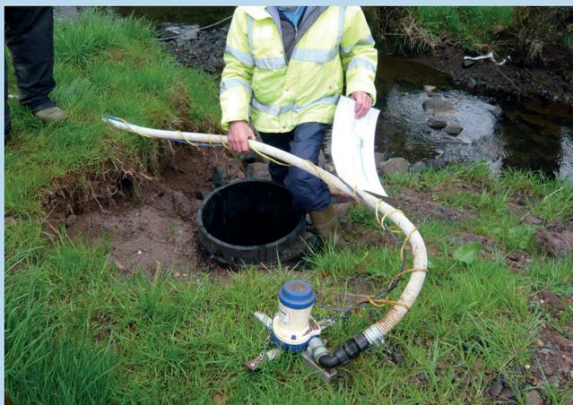
Figure 7: Open abstraction sump chamber for installation of submersible pump.
