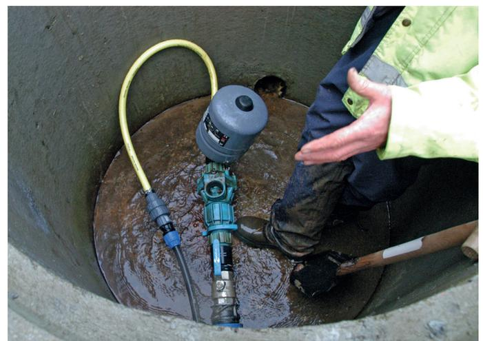
Figure 11. Ram pump within pumping chamber.
