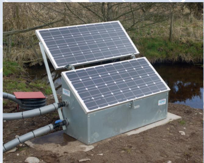
Figure 6: Packaged solar pump unit.
