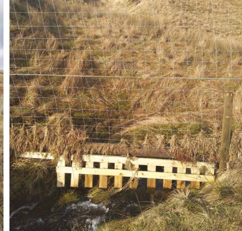
Small water gate.
