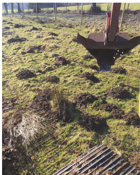
Excavator mounding with a V-shaped bucket.
