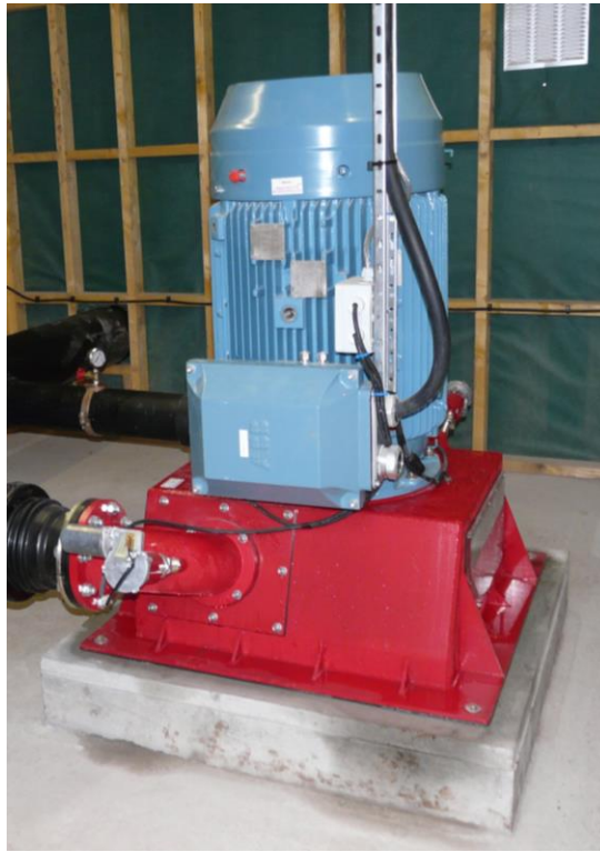
Fig 3 A 50 kW turbine and generator at a high head site.
