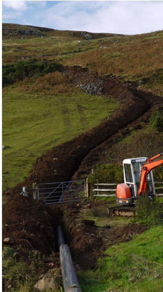
Fig 1 Pipe laying for a small high head hydro scheme
