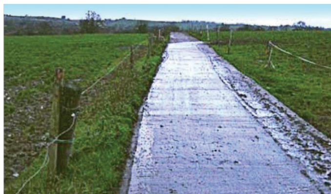
Figure 5. An example of a concrete track. These can be brushed or scraped regularly to keep clean and to prevent the collection of small stones which can cause sole bruising and other injuries.
