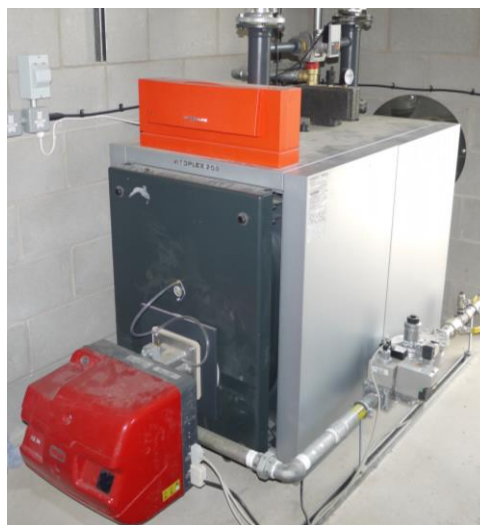
Figure 6: Biogas boiler
