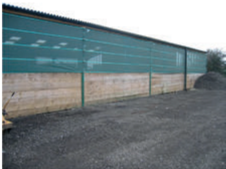
Timber sidewall with ventilated cladding delivers clean fresh air into the building
