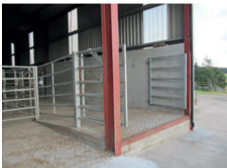
Loading ramp with height suitable for both trailers and HGVs.
