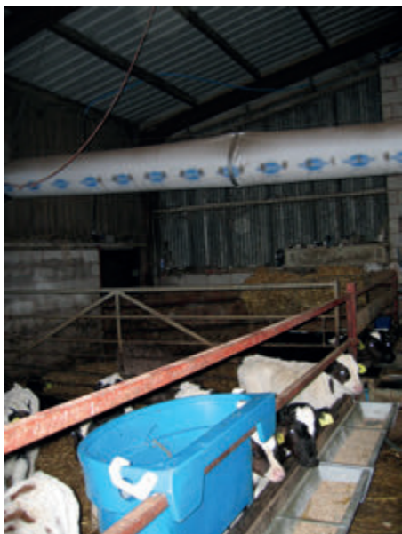
Positive pressure ducting in a calf house
