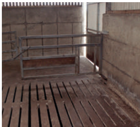
Slatted floor without rubber matting
