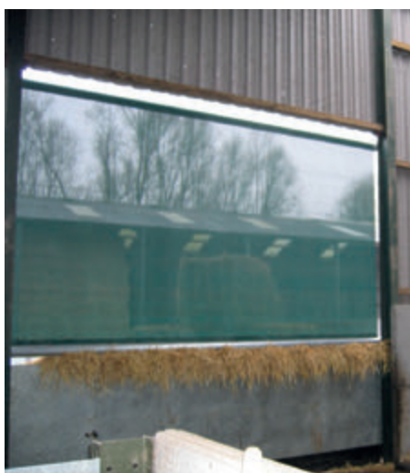
A ventilated roller blind offers protection against draughts
