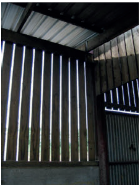
Spaceboard with a simple additional inlet area allows fresh air to enter
