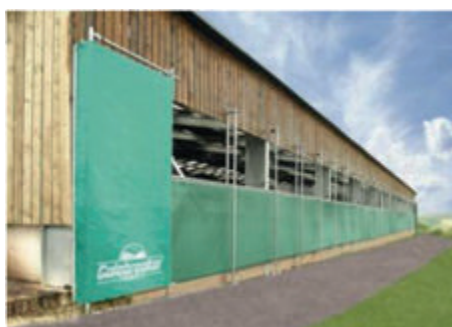
Moving curtains provide flexible inflow of fresh air
