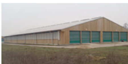
Modern cattle building with a large area of diffuse inlets
