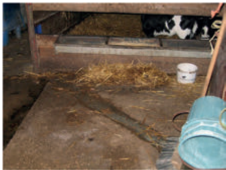
Cutting channels into the existing floor can improve drainage
