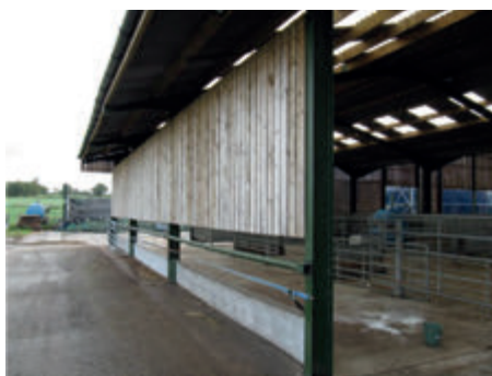
Spaceboard with simple additional inlet area above
